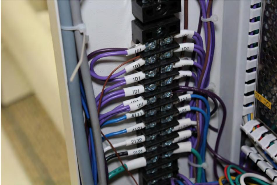
8. The green wire of the 8 conductor cable goes to ground.
